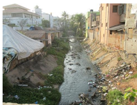
Figure 10-11 Open drains across the city
