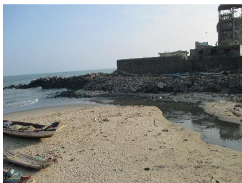
Figure 10-10 Untreated sewage flowing into the sea
