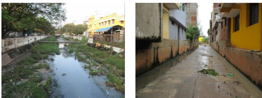
Figure 10-12 Open Drains Running across the Puducherry Planning Area
